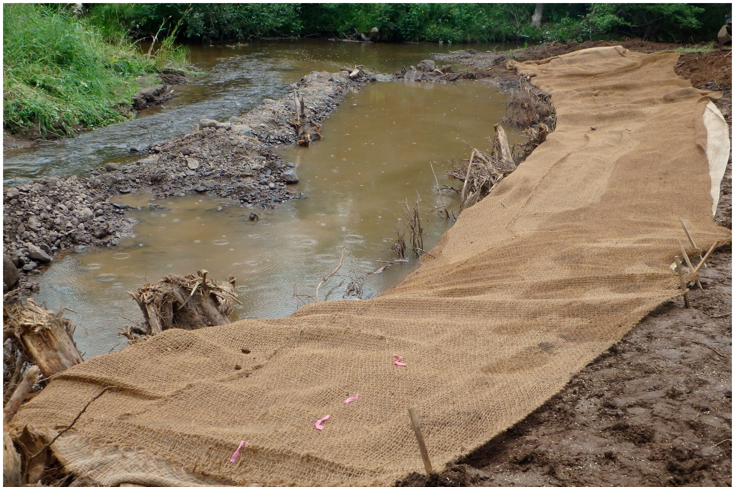
Below, root wads covered with fill, seeded and matted.
