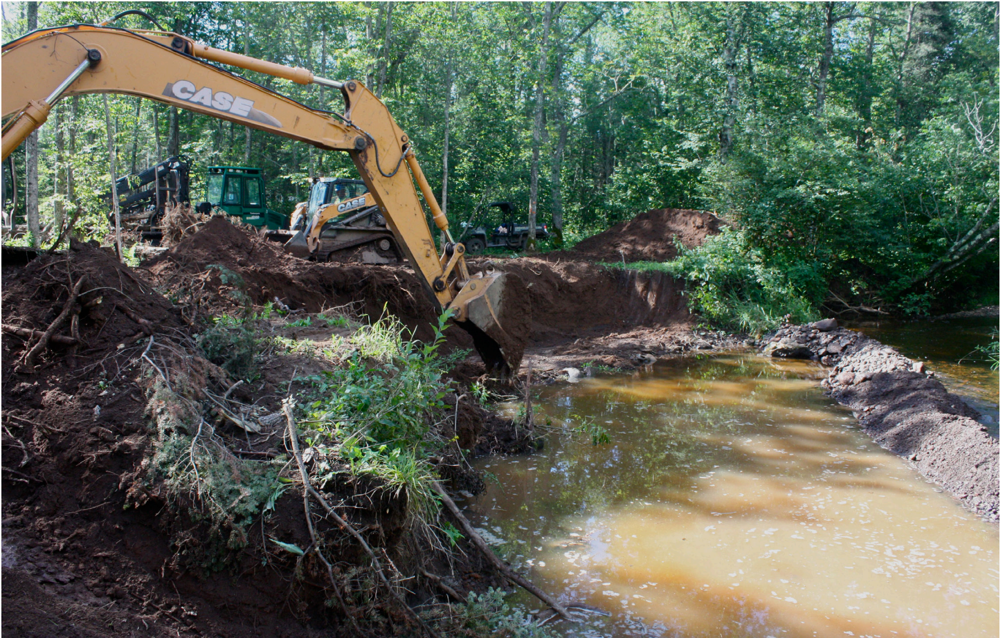
Above, excavating the work area.
