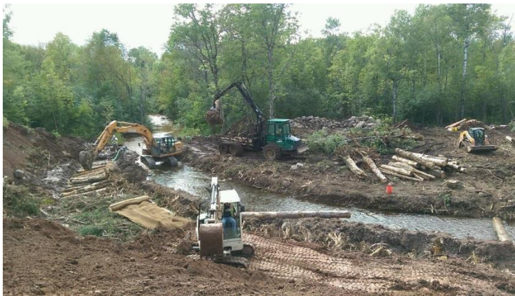
Construction of Reach 12
