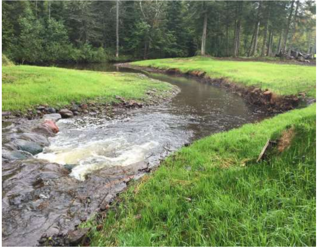
Reach 9 Bank Stabilization and Instream Habitat Project
