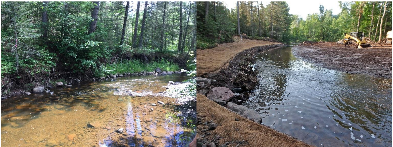
Valentine Reach (constructed in 2017) before and after
