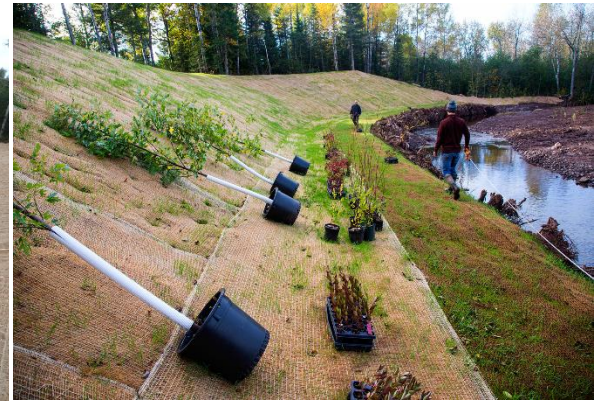
Erosion control and planting of Reach 12
