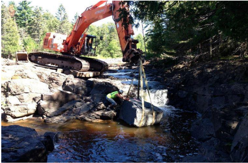
Boulder placement during the construction of the second falls.
