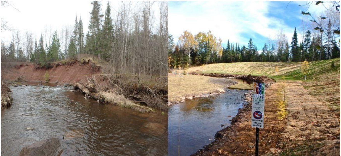
Reach 12 before and after
