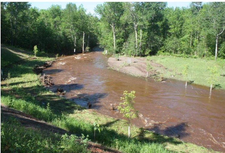
Erosion control and planting of Reach 12
