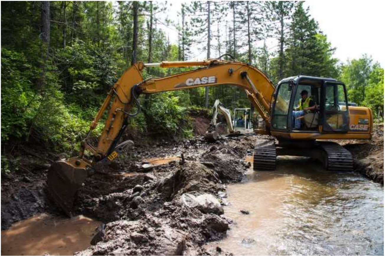
Class CX 160 Class Excavator with Attached Thumb
