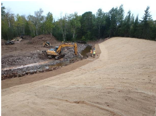
Erosion control and planting of Reach 12
